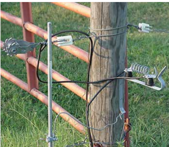
Figure 11-14. MWLA lightning protection.
